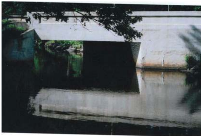
Wheeler Road Bridge
