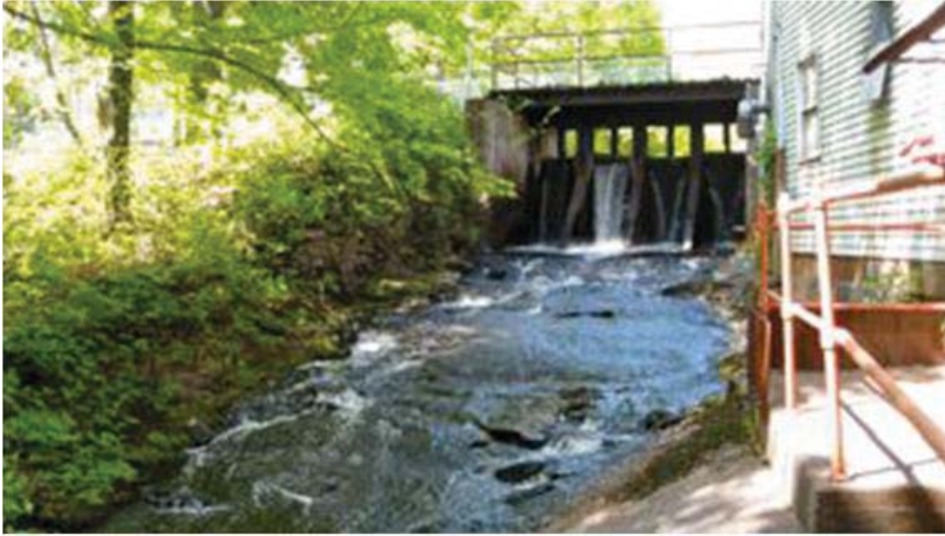
Washington Mills Dam
