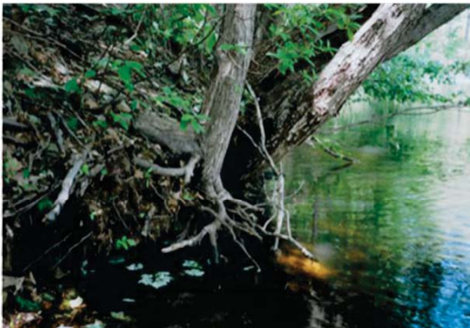
Eroded and undercut embankment
