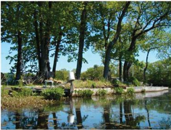
One of several houses with failing retaining walls
