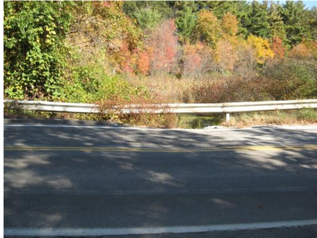
Figure 75 Wrentham Road slumping toward Bungay Brook inlet.
