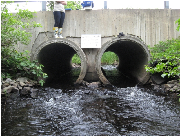
Figure 4 Peters River inlet at Railroad Street.
