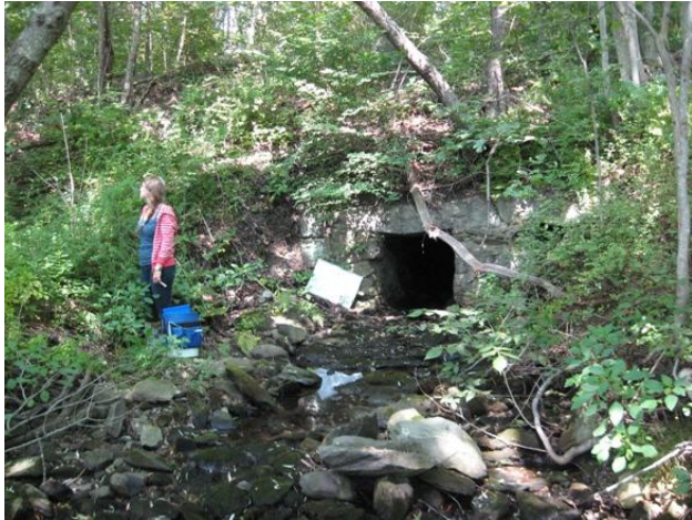
Figure 56 Arnolds Brook inlet at SNETT.
