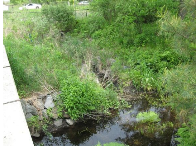
Figure 65 Flow from detention basin adjacent to Arnolds Brook at Pulaski Blvd/Deer Run Road.
