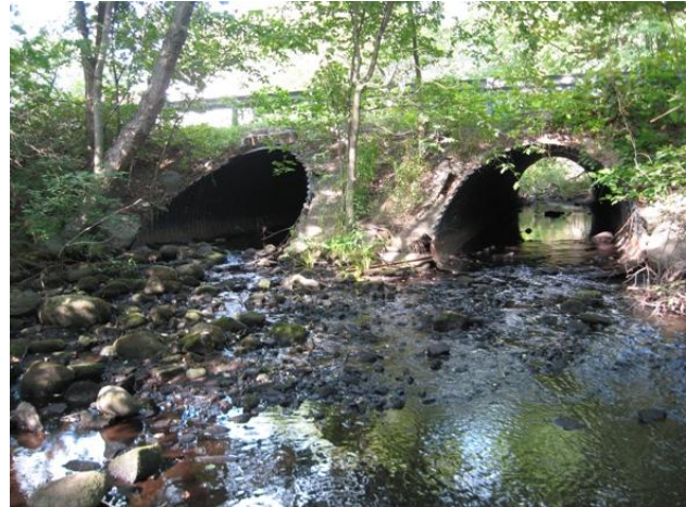
Figure 19 Peters River outlet at Paine Street.
