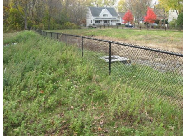
Figure 23 Detention pond adjacent to Peters River at Paine St. - Photo 3.
