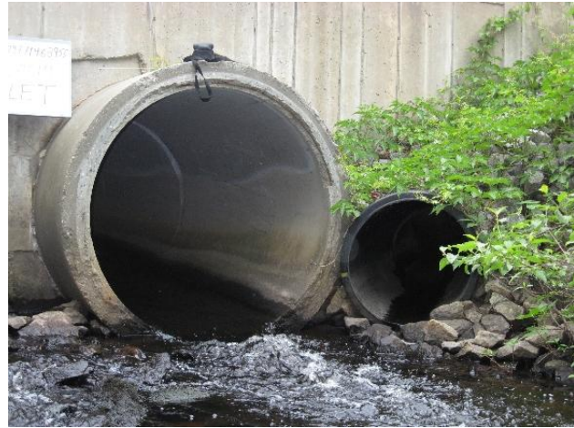
Figure 5 Peters River outlet at Railroad Street.
