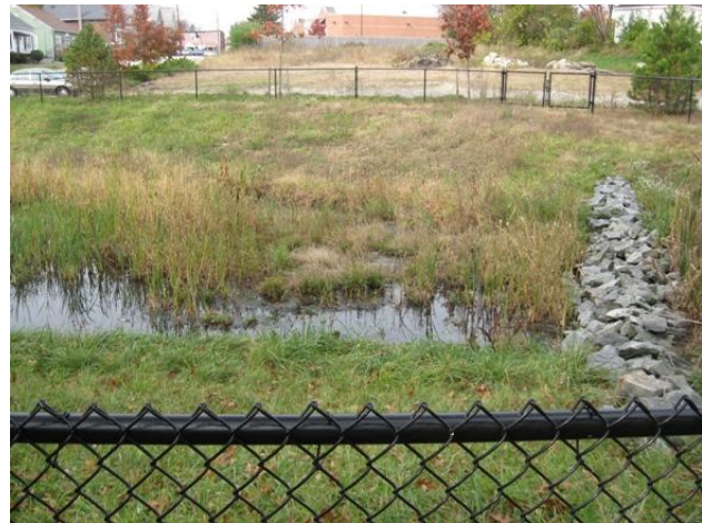
Figure 21 Detention pond adjacent to Peters River at Paine St. - Photo 1.
