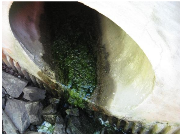
Figure 11 Outflow adjacent to inlet at Pulaski Blvd.
