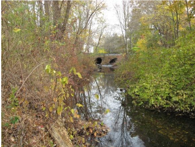
Figure 27 Upstream from detention pond outlet
