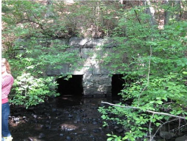
Figure 2 Culvert under the Southern New England Trunk Trail.
