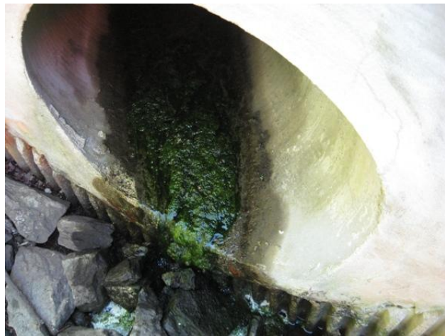
Figure 9 Outflow adjacent to inlet at Pulaski Blvd.
