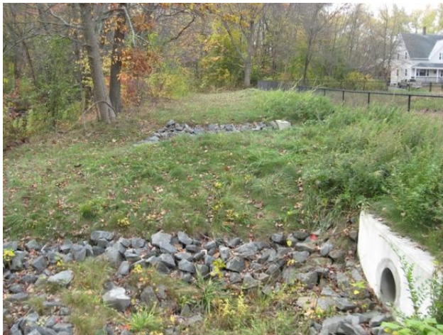
Figure 24 Detention pond adjacent to Peters River at Paine St. - Photo 4.
