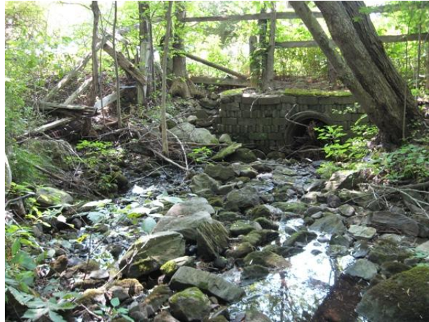
Figure 57 Arnolds Brook downstream from SNETT. Inlet to underground portion of brook.
