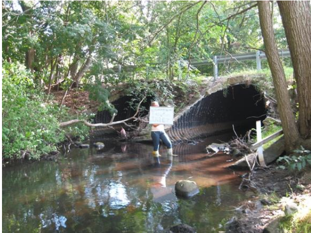
Figure 18 Peters River inlet at Paine Street.
