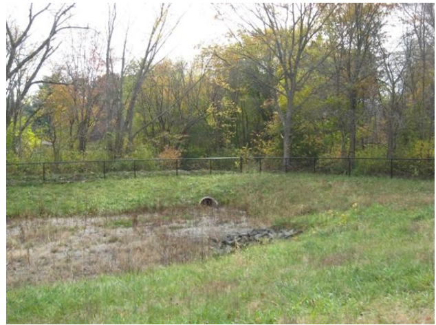
Figure 25 Detention pond adjacent to Peters River at Paine St. - Photo 5.
