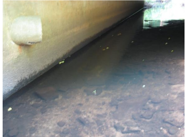
Figure 15 Outflow at Wrentham Road causing scour.
