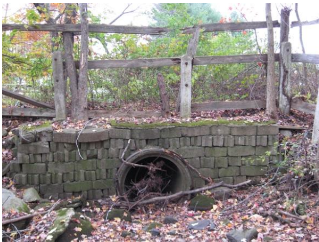
Figure 58 Inlet to underground portion of Arnolds Brook.
