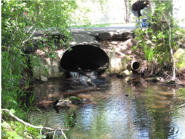
Figure 60 Arnolds Brook outlet at Lizotte Drive.
