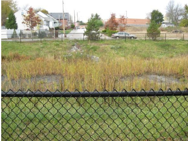
Figure 22 Detention pond adjacent to Peters River at Paine St. - Photo 2.
