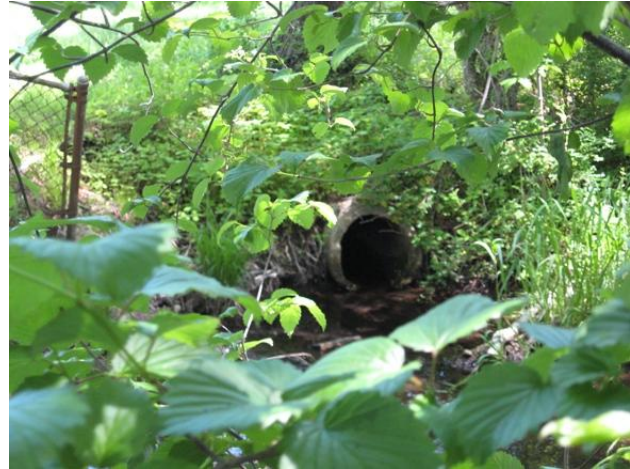
Figure 61 Outflow from adjacent property at Lizotte Drive.
