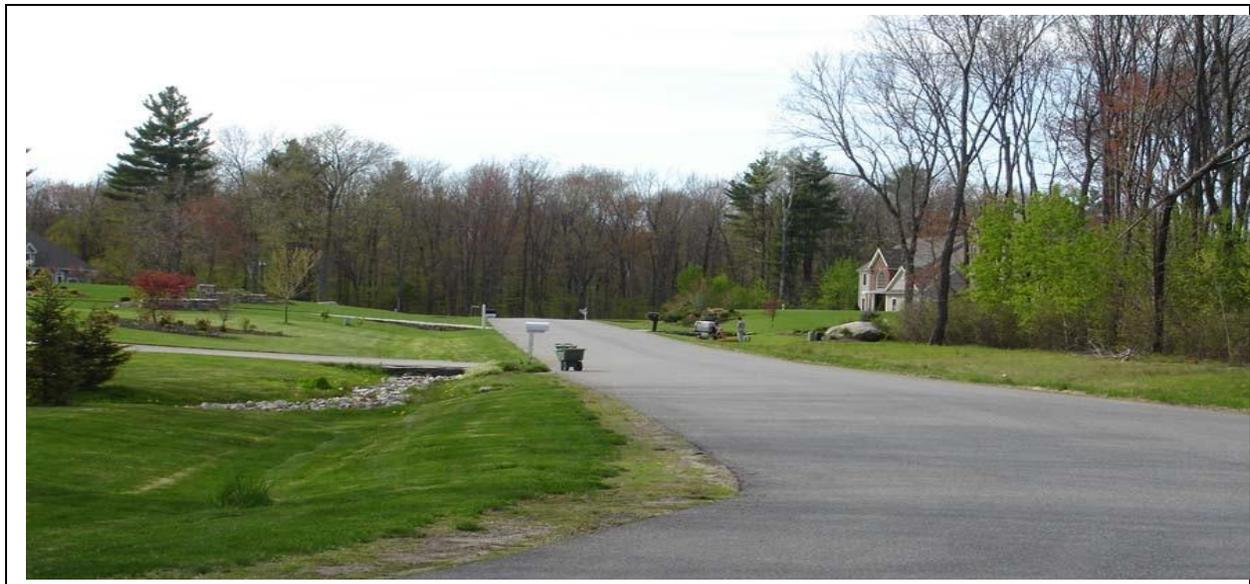
Rebekah Drive in Sutton is a good example of “country drainage”. It is a small residential cul-de-sac, with narrow widths of pavement, no sidewalks, and grass swales to handle stormwater. No curbs, no catch basins.
