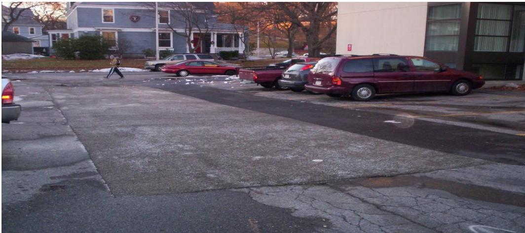
A section of the parking lot at WPI in Worcester, MA has been paved with porous concrete. The melting snow goes right through the concrete!
